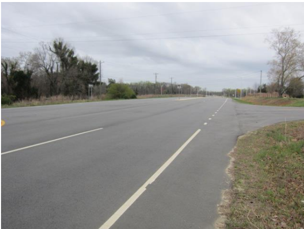
View Looking South Along Germanton Road
