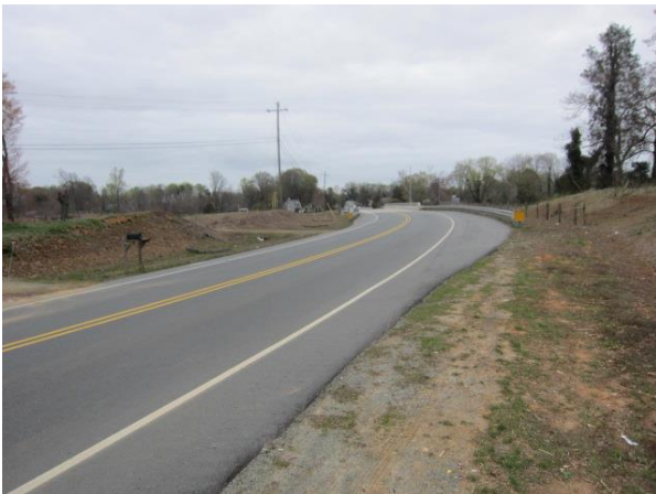
View Looking East Along Old Hollow Road
