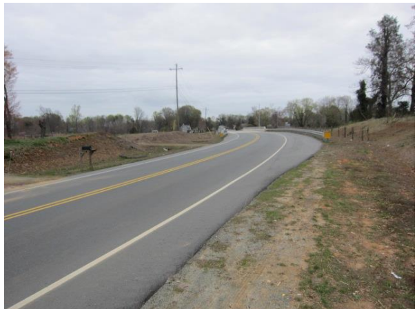
View Looking West Along Old Hollow Road
