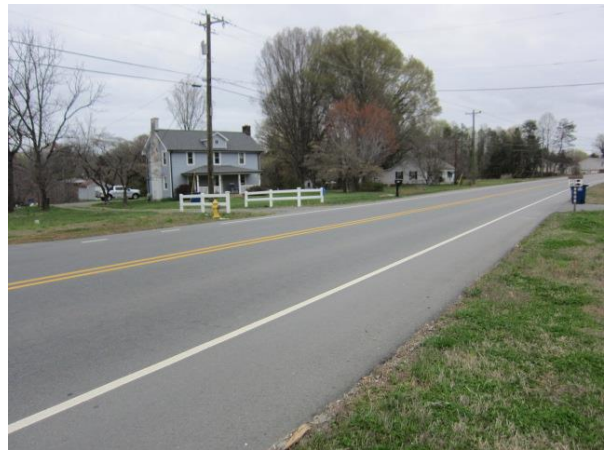
View Looking West Along Old Hollow Road
