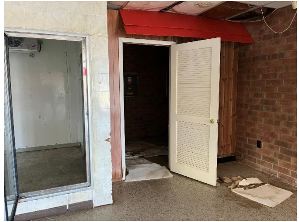
Interior view, storage room
