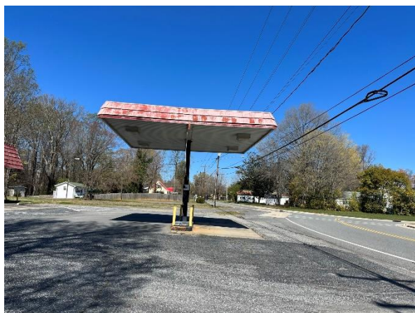
View of canopy and area of the easement
