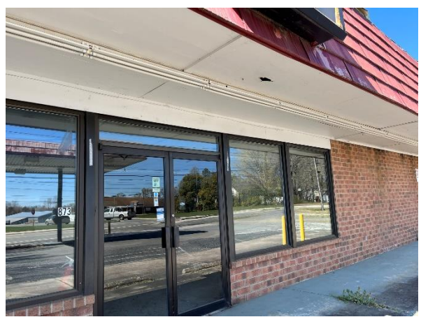
Front storefront view
