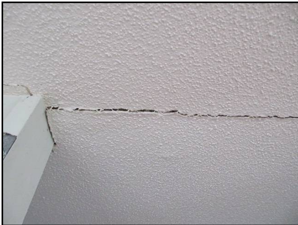
10. Cracked Ceiling Drywall
