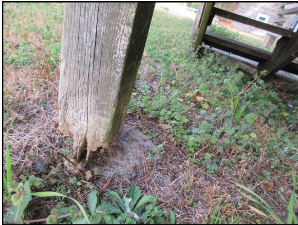
14. Rotted Deck Piling
