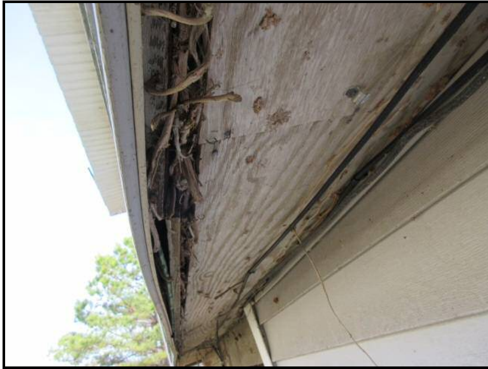
17. Damaged Soffit
