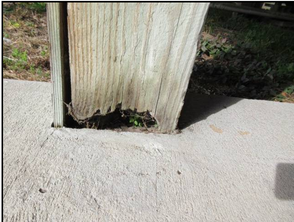
18. Damaged Piling
