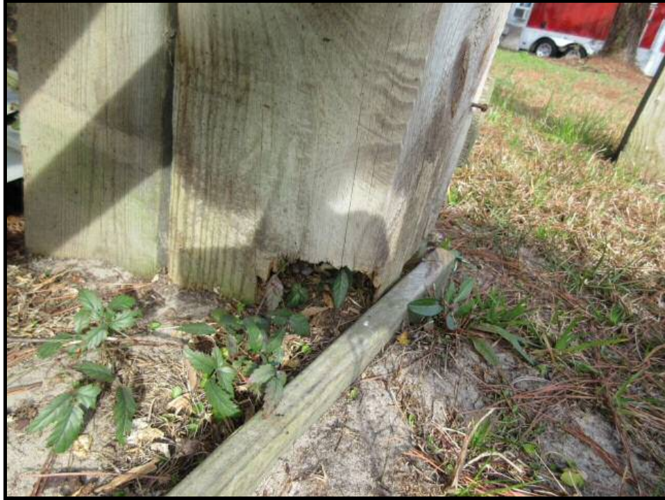
13. Rotted Piling with Sistered Piling
